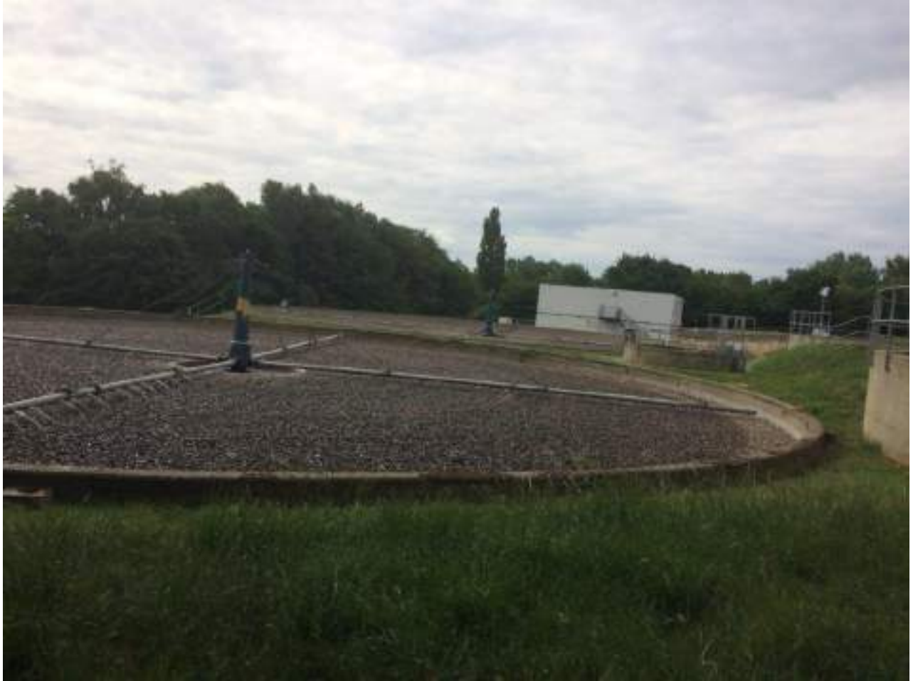
Photograph 15 – An active sewage treatment plant found to the south-east of the site
