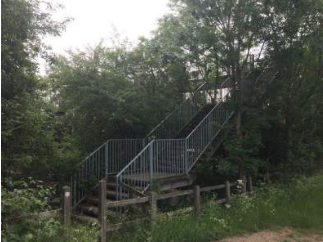
Photograph 11 – Footbridge across the A10.
